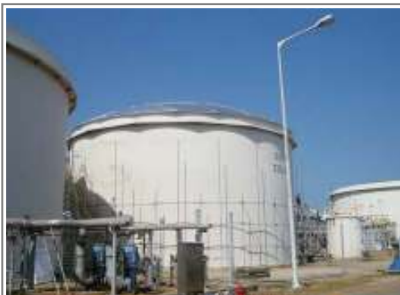
Hyundai Petrochemical complex three(3) x 18m Al. Dome construction site at Daesan, Korea
