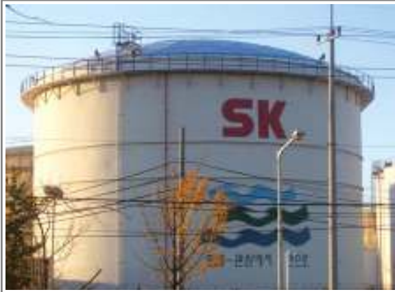
SK Oil Storage Tank AL. Dome Cover ( \varnothing 25m) in Incheon Port City. 2004.01
