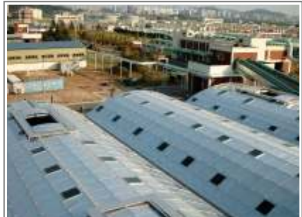
Seonam WWTP AL. Dome Cover (24m,20m,20m x 59m) in Seoul City
