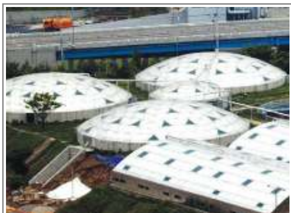
Sunghwan WWTP AL. Flat Cover in ChungCheong, Province in Korea
