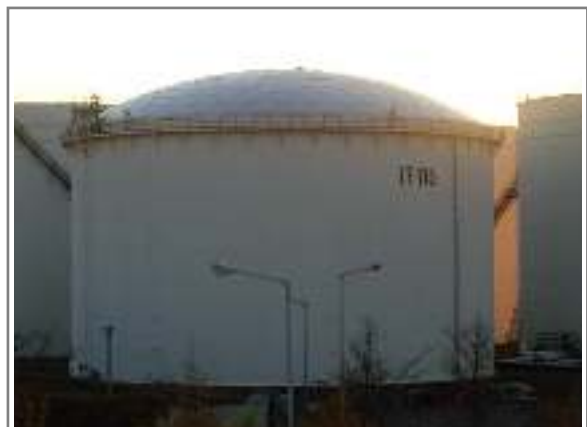
SK Oil Storage Tank AL. Dome Cover ( \varnothing 34.5m) in Incheon City
