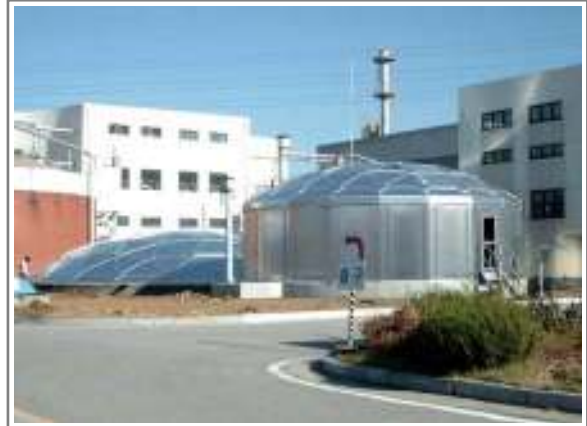
WWTP AL. Dome Cover for Biological Treatment Ponds( \phi 15m, \phi 10m, 6sets) in Guri City, Korea
