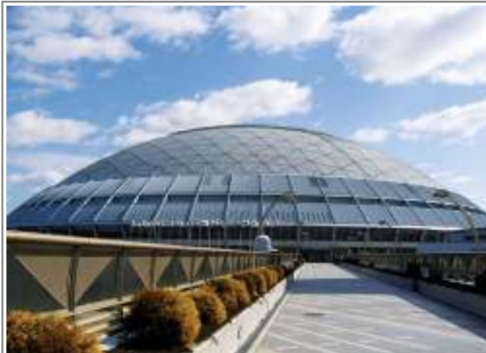
Dome for Sport Stadium
