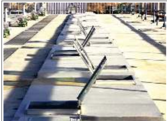
Special Surface Treated AL. Flat Cover for Kimpo City WWTP in Korea
