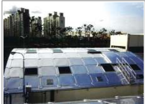
Samsung Electronics Suwon Factory WWTP 15mx20m in Suwon, Korea. 2003
