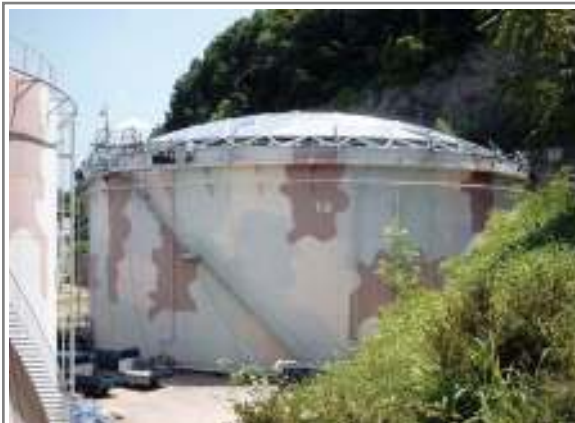
Al. Dome for Grip Hoist erection site due to mountain area of oil storage tanks.
