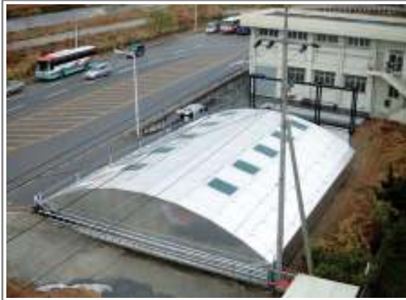
Aluminum Dome Cover for WWTP Uam Pump Station in Chung-Ju City (16m x 20m)
