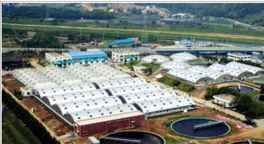
WB has installed many different types of Al. Dome Roofs at Guri City WWTP. Total twenty six(26) AL. Dome Covers built from year 2003 to 2004
