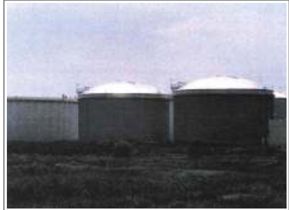
Hyundai oil Refinery's BTX Storage Tank AL. Dome Cover ( \varnothing 40m, \varnothing 28m) in Incheon Port City
