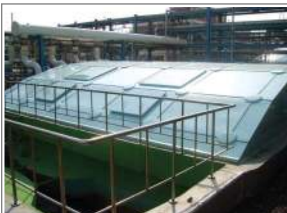
AL.Flat Cover for Ulsan City WWTP, Ulsan City is One of the Most Industrial City in Korea
