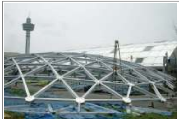
Assembling Main Frame
