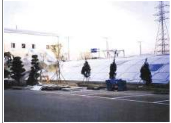
WWTP AL. Dome Cover, Hopper Room & Conveyor Systems (22m x 30m) in Guri City, 2001
