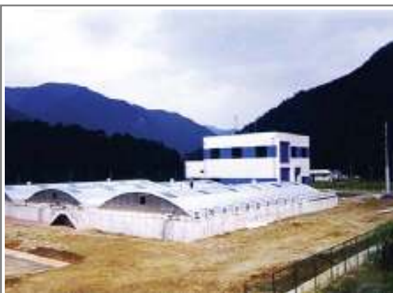
Dogae city WWTP AL. Dome Cover (14m x 32.5m, 3set) in KangWon Province
