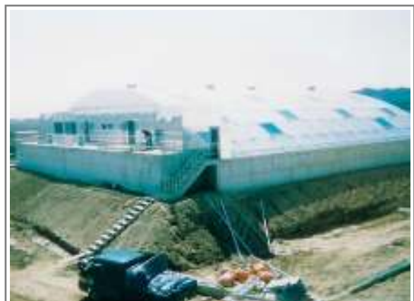
Hameol STP AL. Dome Cover (29m x 30m) in Jeollabuk Province
